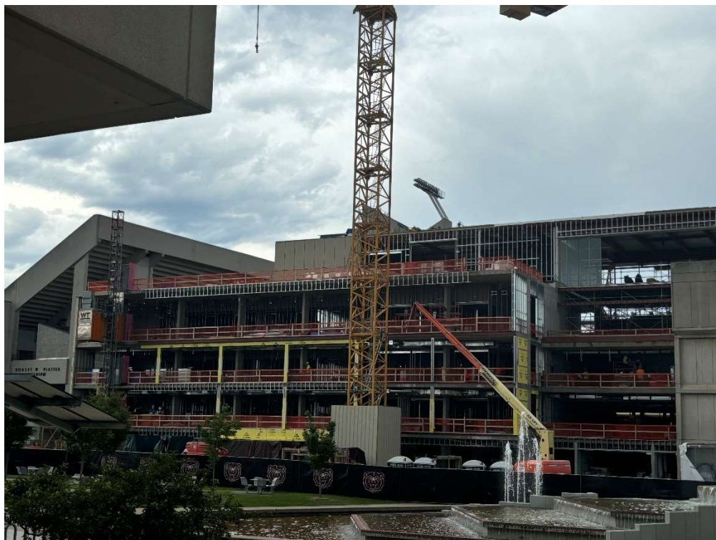
(Construction of the Roy Blunt Hall renovation and addition)
