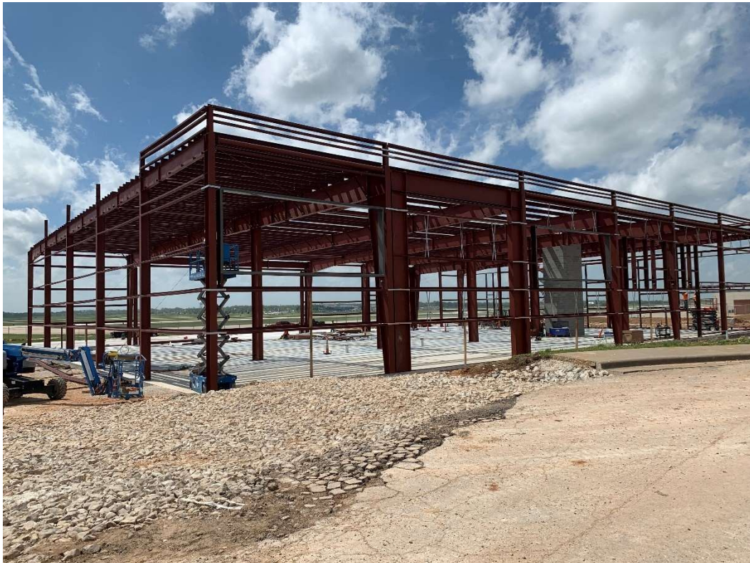
(The skeleton of the facility in early 2024)
